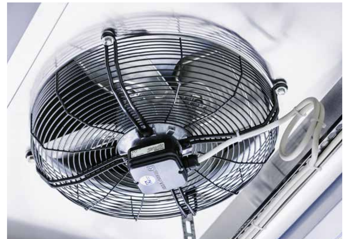
AIR COOLED CONDENSERS HELP REFRIGERATE THE COLD STORAGE ROOM IN A FOOD STORE IN THE NEW EMPORIA SHOPPING MALL IN MALMÖ.
